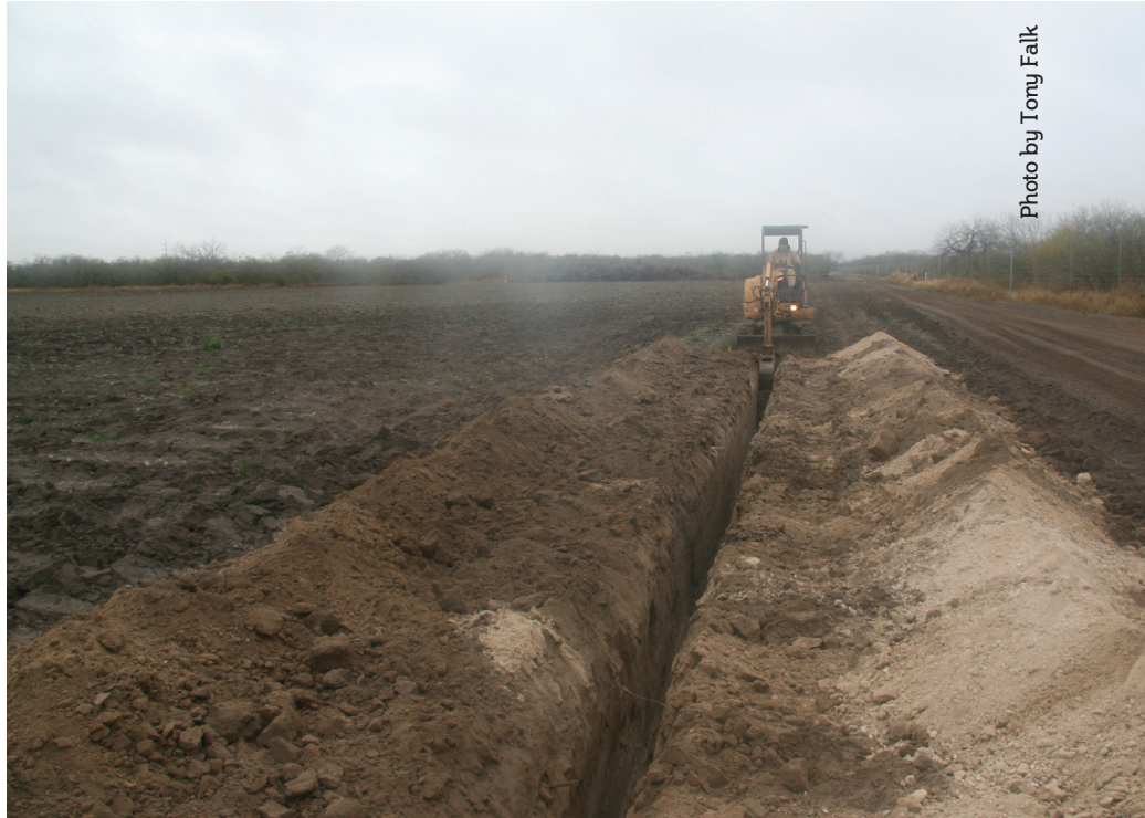
When trenches for pipelines are dug, we recommend “double ditching.” This is a method in which the immediate topsoil is removed to one side, the trench is then dug, and soil stored to keep the topsoil and the subsoil separate. Following construction, the layers are put back in the same way they came out to prevent subsoil from being mixed with the topsoil and causing problems such as high salinity.
