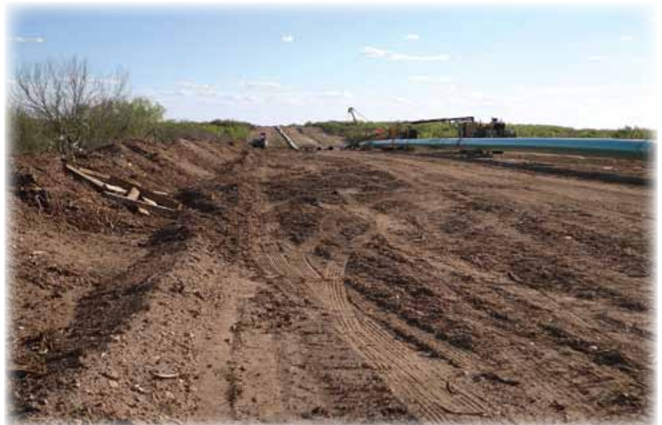
Eagle Ford Shale pipeline installation.
