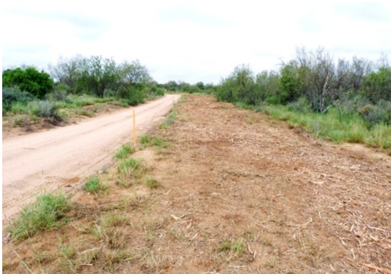
Figure 2. Pipeline under construction that parallels an existing ranch road.
