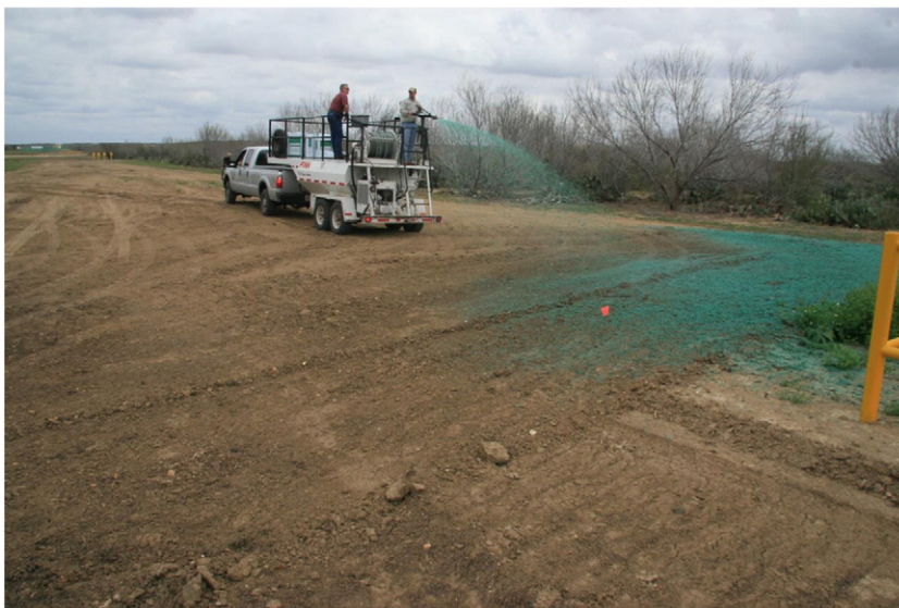
Figure 3. Hydroseeder. Photo by Forrest Smith.
